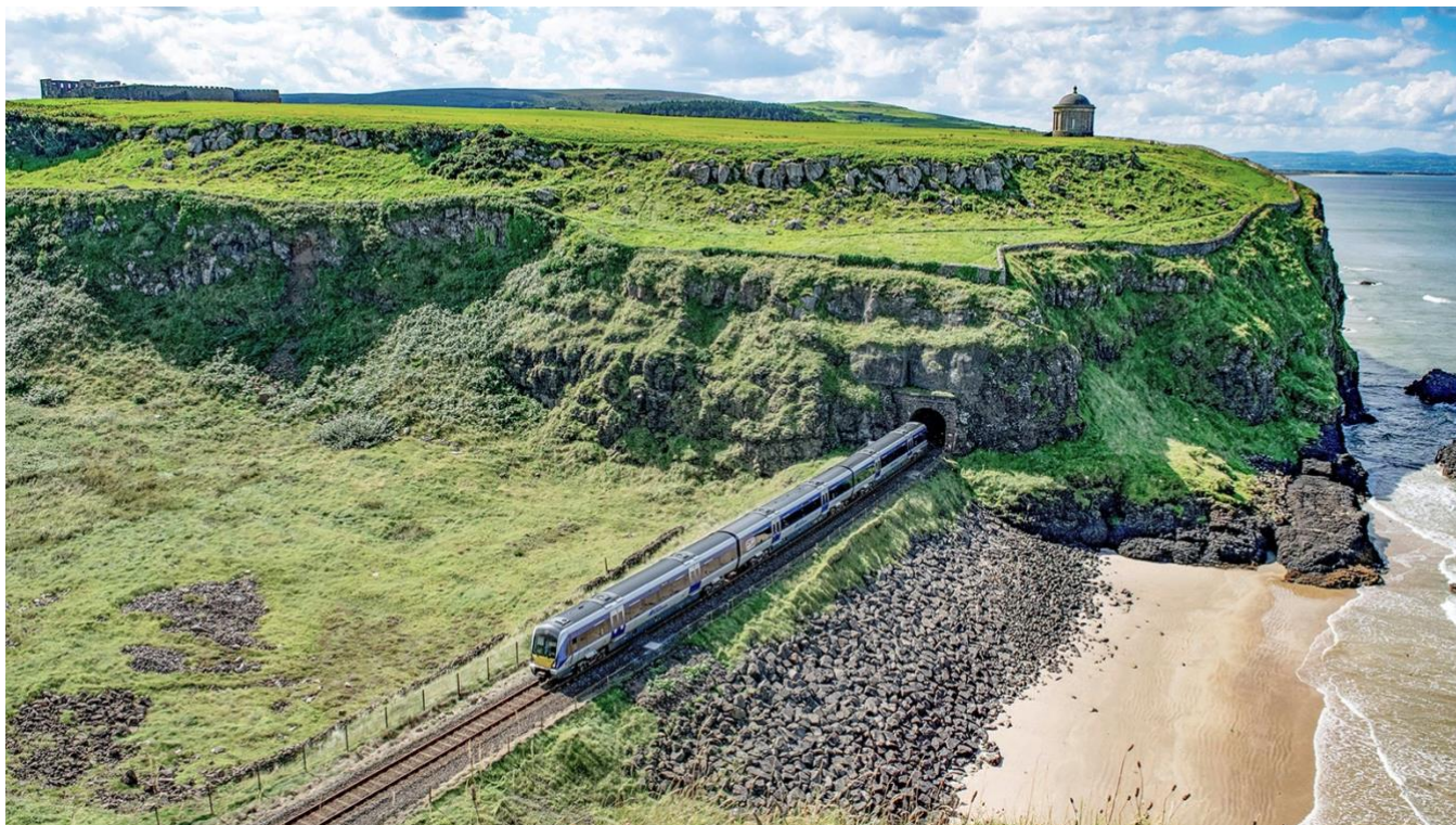
Train passing through tunnel along the north-west coast of Northern Ireland. © Eoin McConnell www.eoinmcconnell.com
